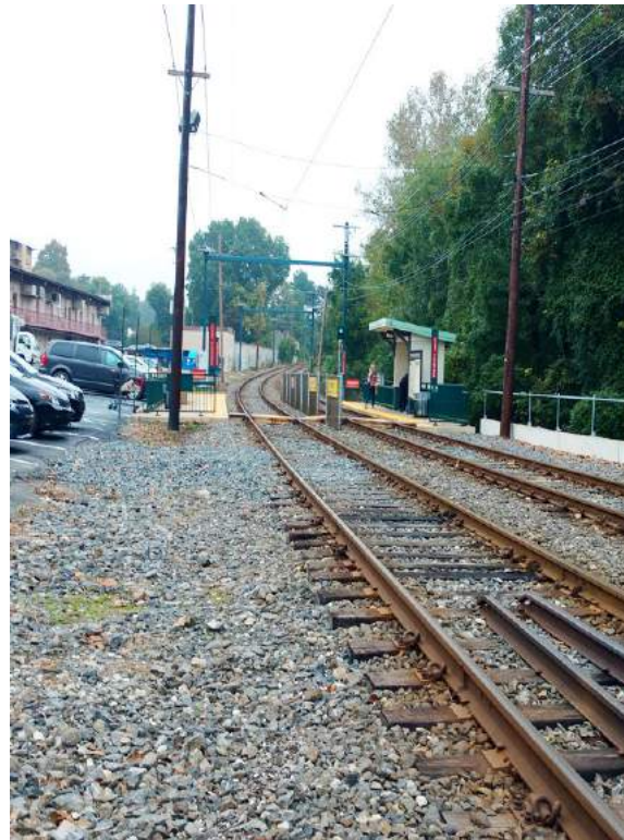
Drexeline Septa Station with existing pedestrian crossing
