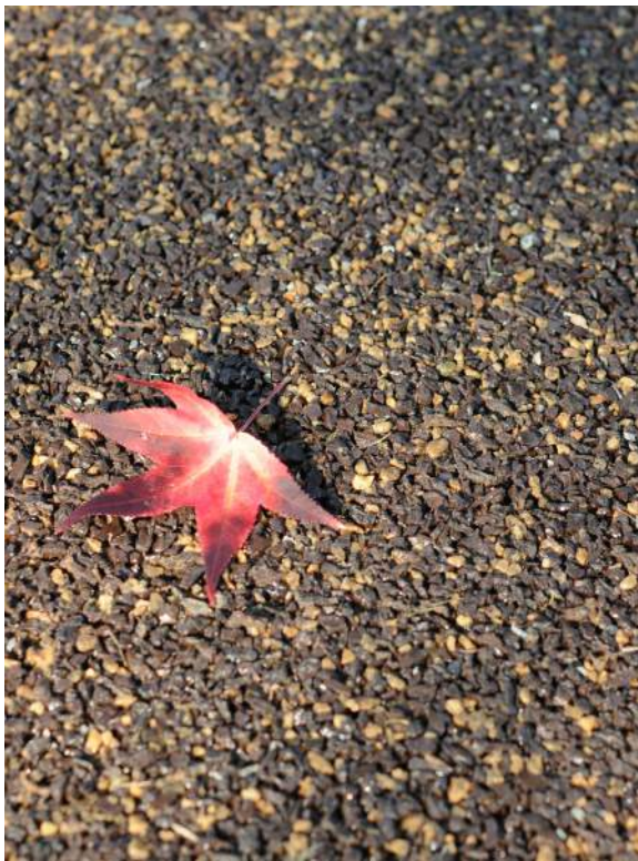
Pervious Pavement may be a consideration in areas where it is desirable to improve water quality through infiltration. Photo shows close up of a rubber-granite pervious pavement.
