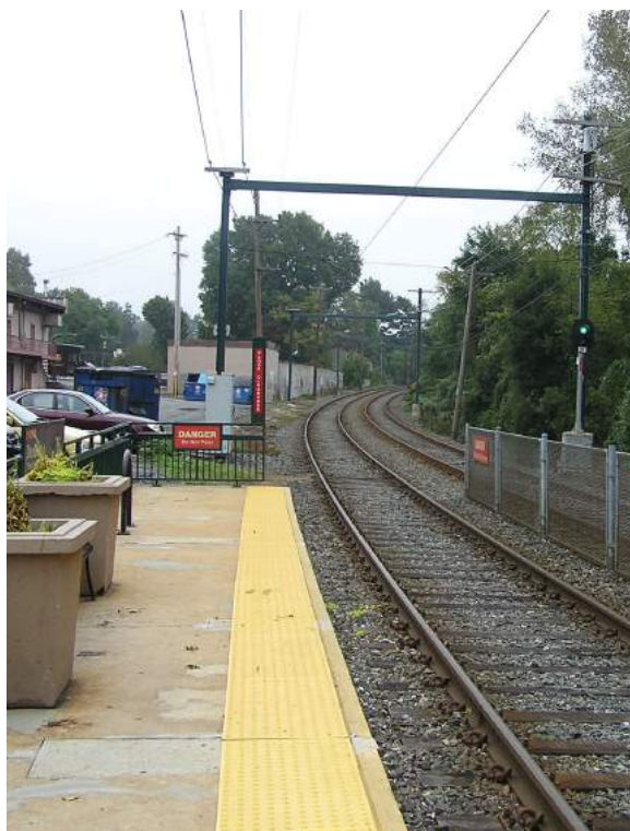
Septa station and tracks looking north
