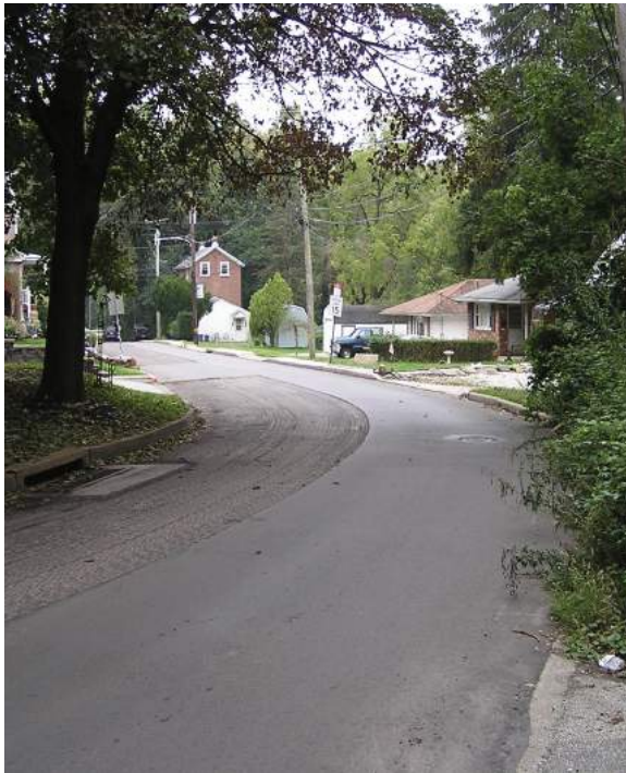
Incomplete Sidewalks on Bloomfield Avenue Looking down towards Huey Park from entrance to Drexelbrook Community
