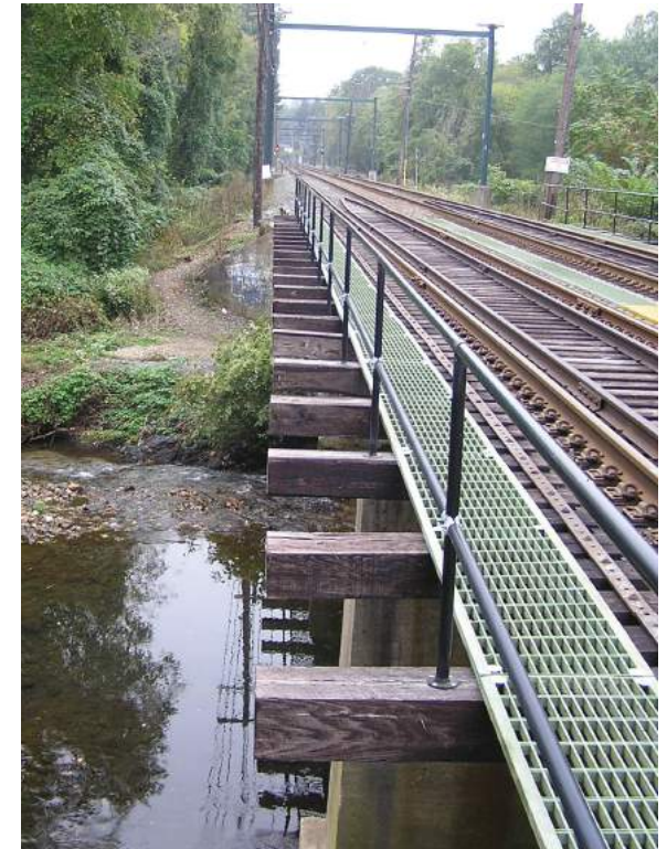
Septa lines and bridge over Darby Creek looking south from Septa station
