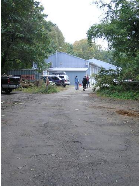
Service road and proposed trail route behind Drexelbrook Community and looking towards maintenance building
