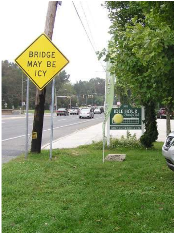
Incomplete sidewalk on US Route 1 looking southwest towards the bridge scheduled for replacement and the tennis club
