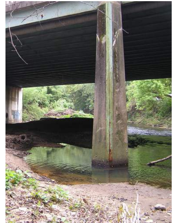
Under the US Route 1 bridge scheduled for replacement and potential trail route. Would avoid US Route 1 - State Road Crossing
