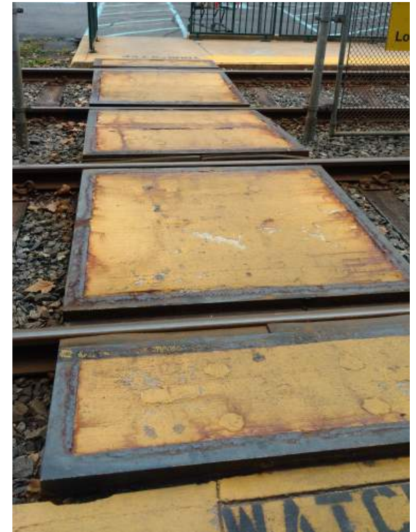
Existing crossing at Drexeline Septa Station
